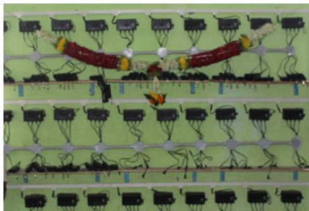
Muthur Charging station
