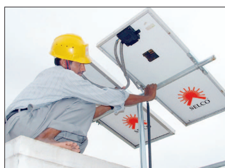
ALL SET: A technician installs a solar panel
